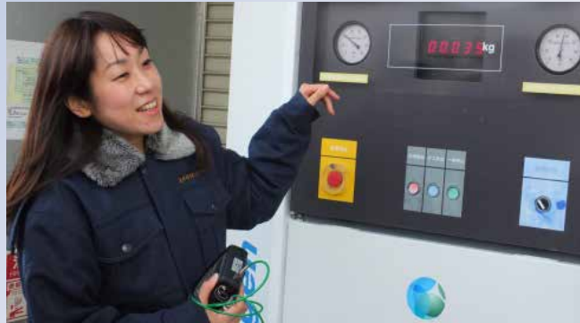
Figure 6: Using leak detectors is not part of the refilling procedure in other parts of the world. Apart from this there is no difference.
