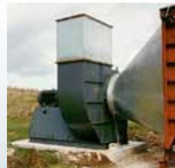
The end plate and the centrifugal fan
